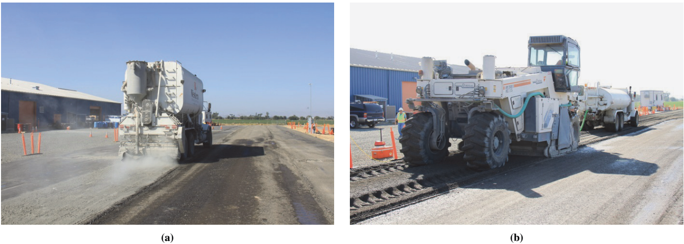
FIGURE 1 FDR-PC test track construction: (a) spreading cement and (b) water addition and mixing.
