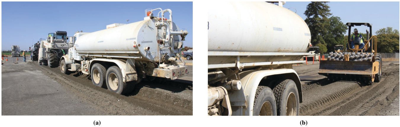
FIGURE 1 FDR-FA test track construction.
