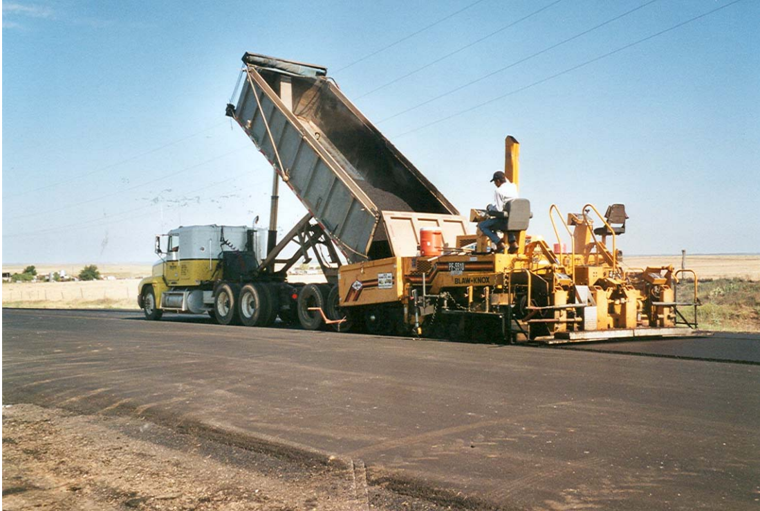
FIGURE 13 Placement of HMA overlay on US 412 Beaver, County.
