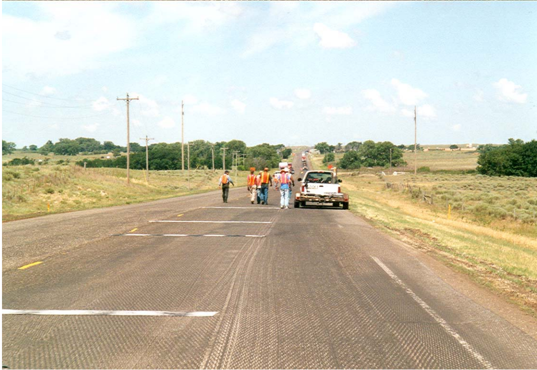
Figure 19 Installation of precoated fabric membrane strips.
