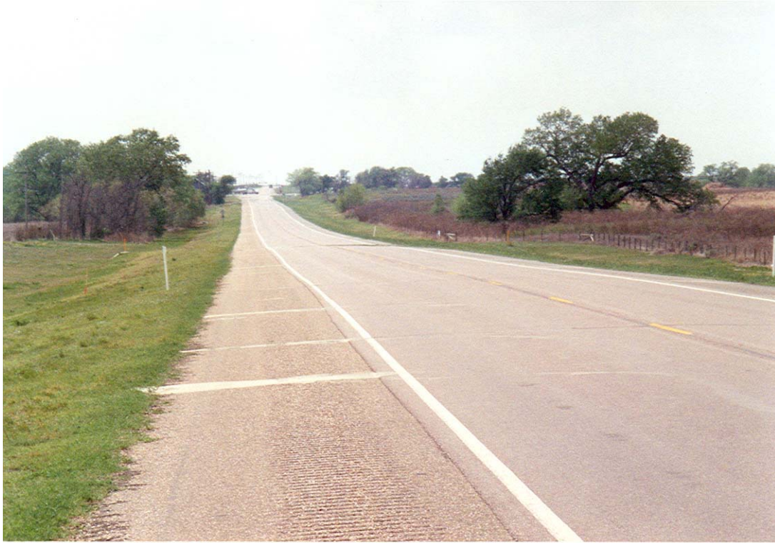
FIGURE 15 US 412 Harper, County after slurry crack injection.
