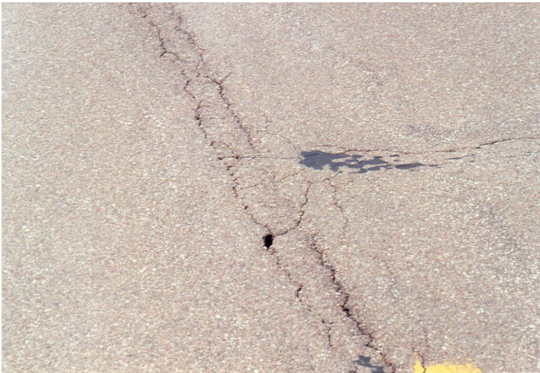
FIGURE 14 Typical distress on US-412 Harper, County.
