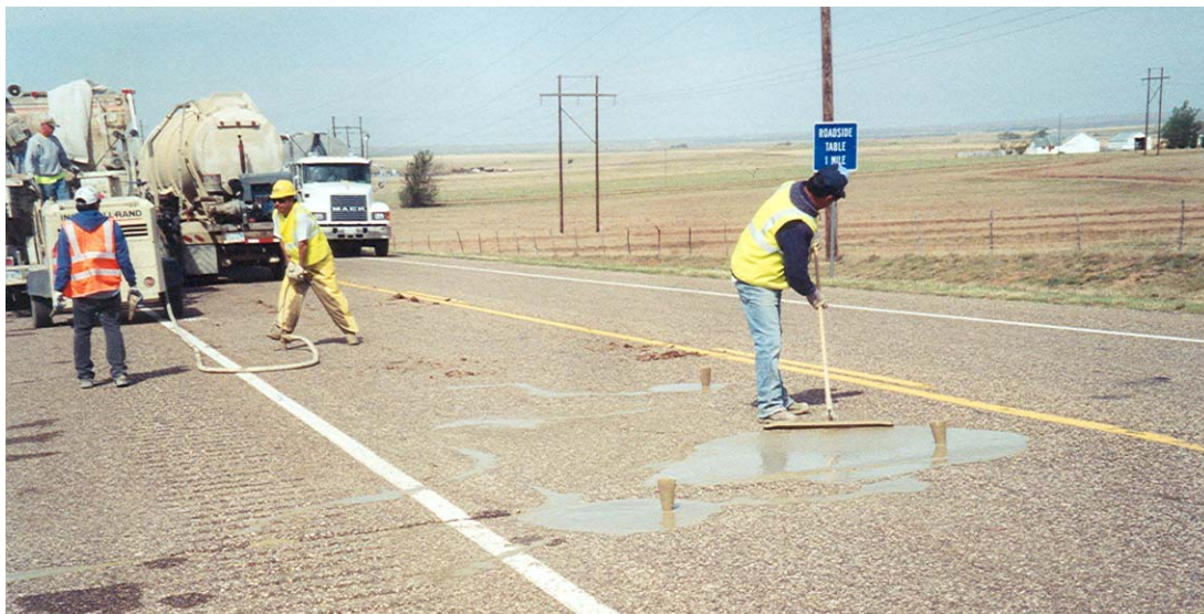
FIGURE 7 Fly ash slurry crack injection on US 412.
