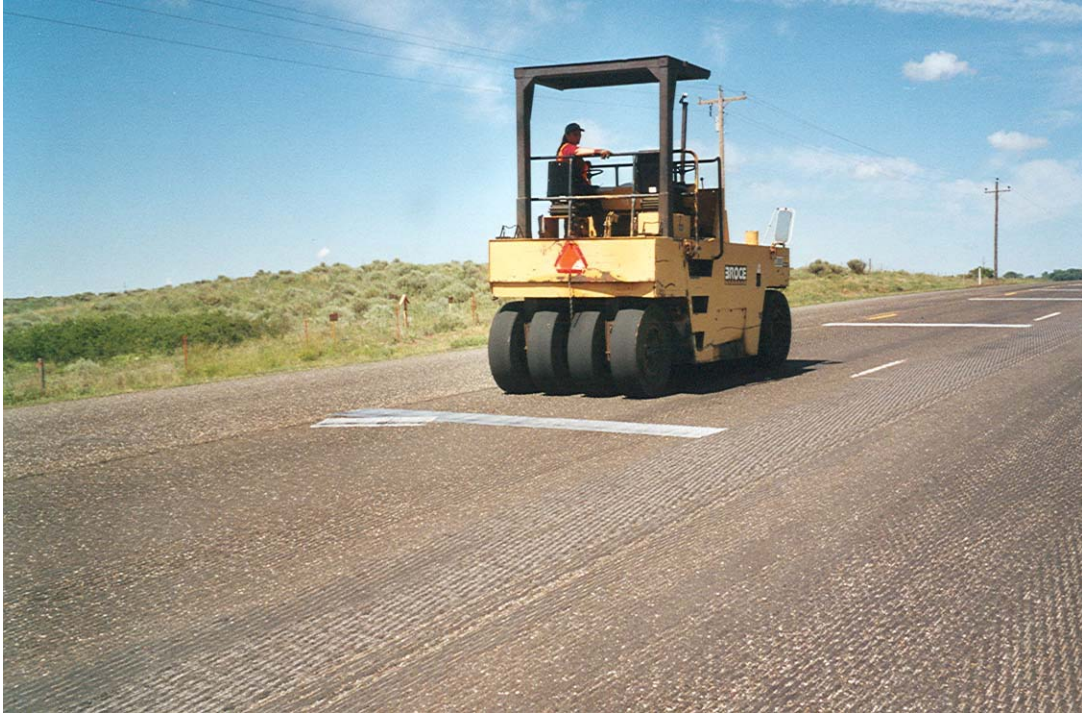
FIGURE 17 Seating pre-coated fabric membrane strip with pneumatic roller.
