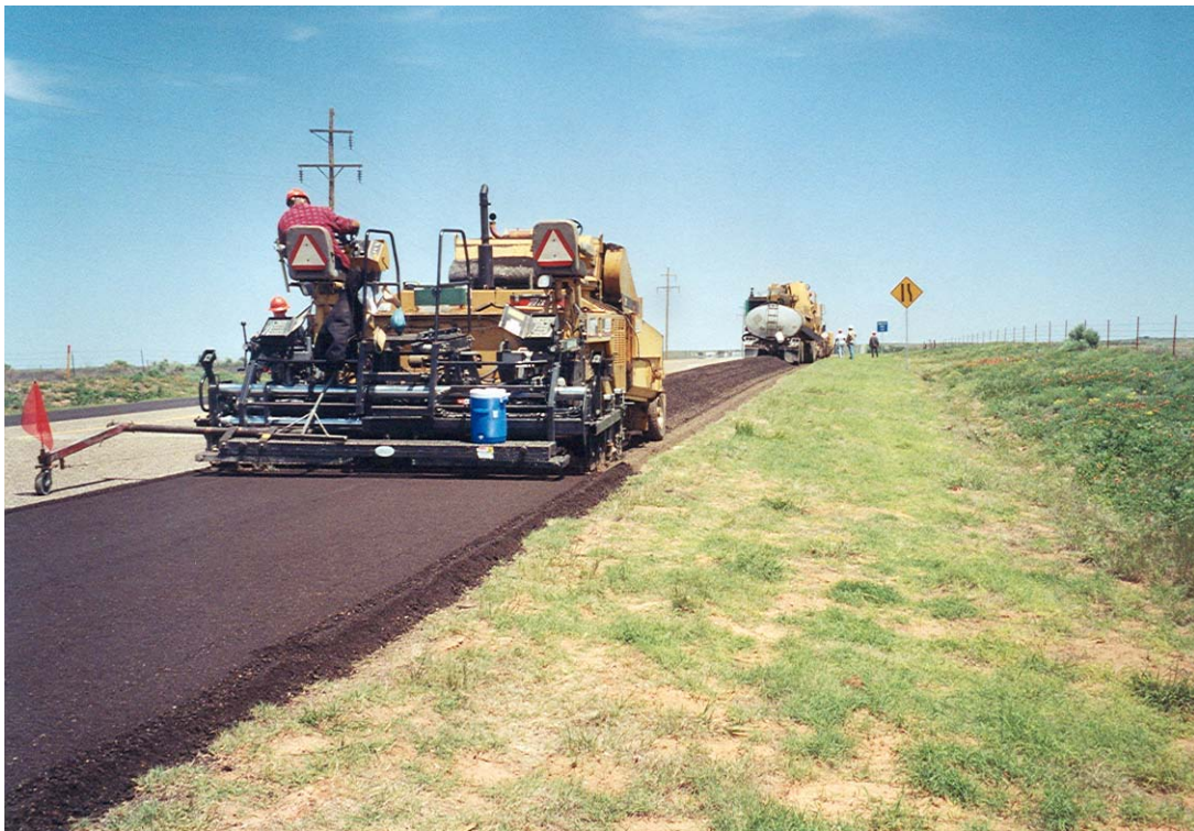
FIGURE 12 Laydown of CIR mixture.
