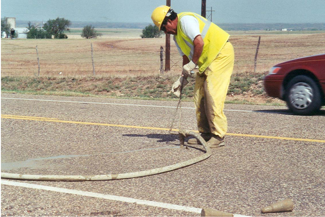
FIGURE 9 Pressure injecting transverse cracks with slurry.
