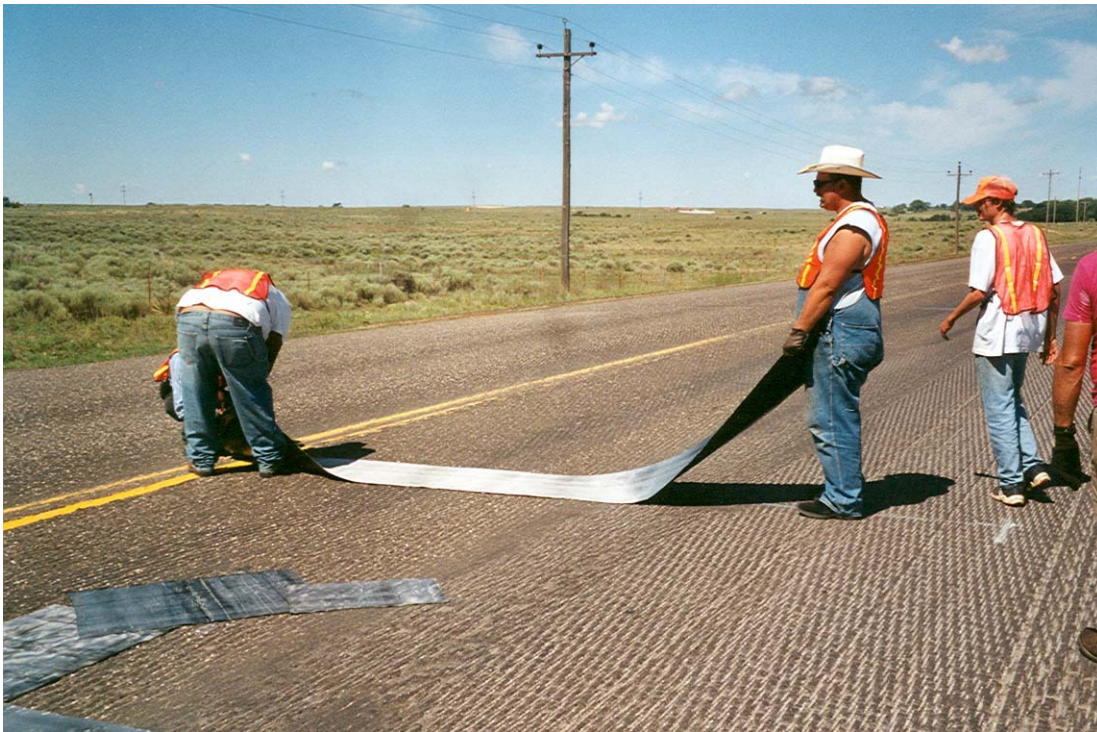
FIGURE 16 Installation of pre-coated fabric membrane strip.
