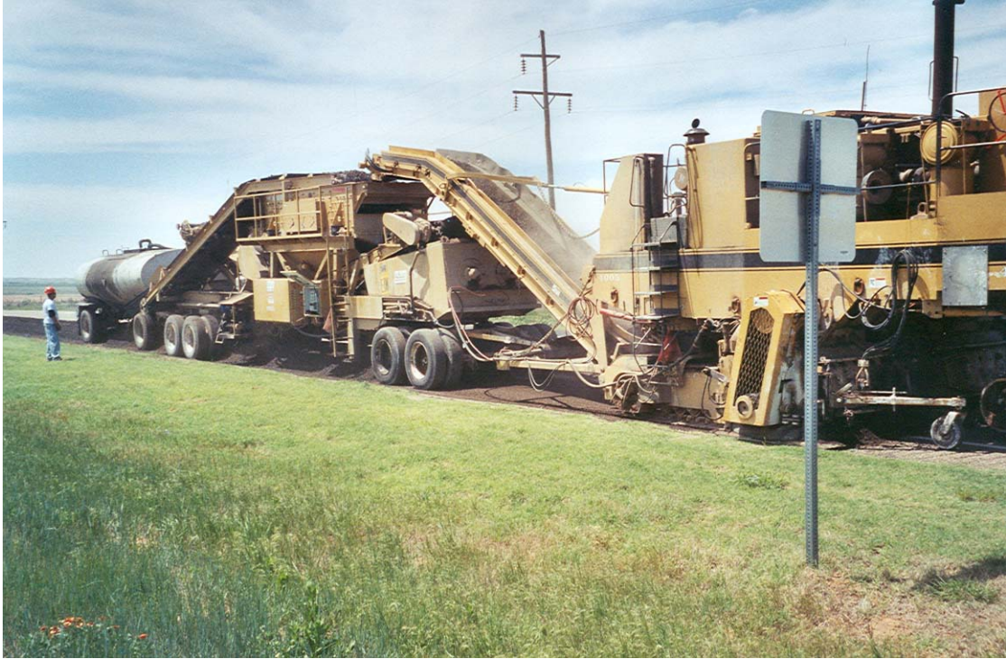
FIGURE 11 Cold recycling US 412 with multi-unit CIR train.
