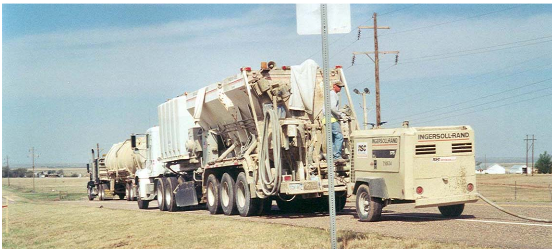
FIGURE 8 Slurry injection equipment.
