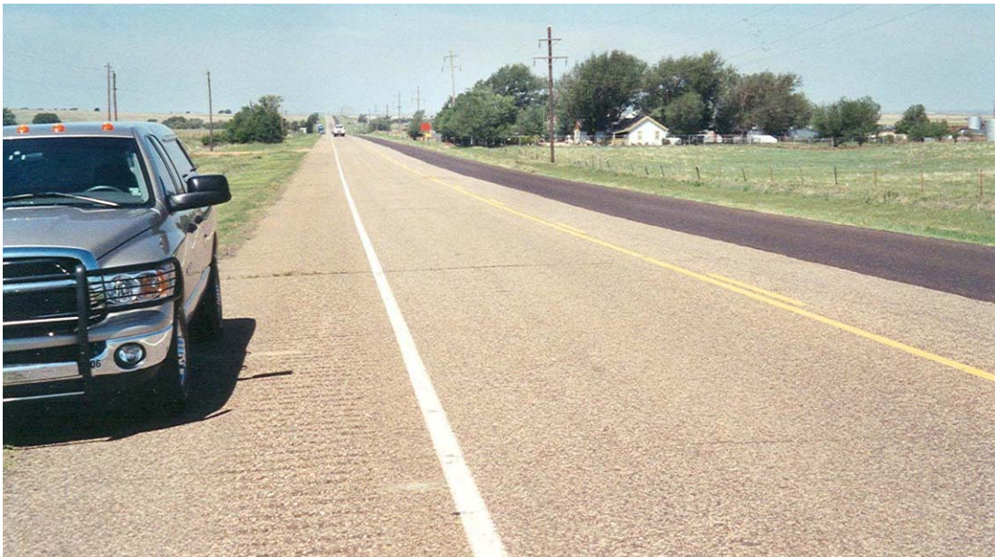
FIGURE 6 US 412 prior to CIR rehabilitation.
